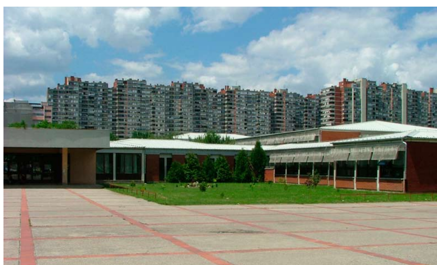
Primary school building located in the park of Travno
